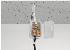
Pendant light connection in a suspended ceiling
