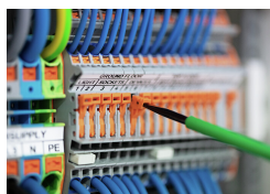
Pivoting a knife disconnect.
